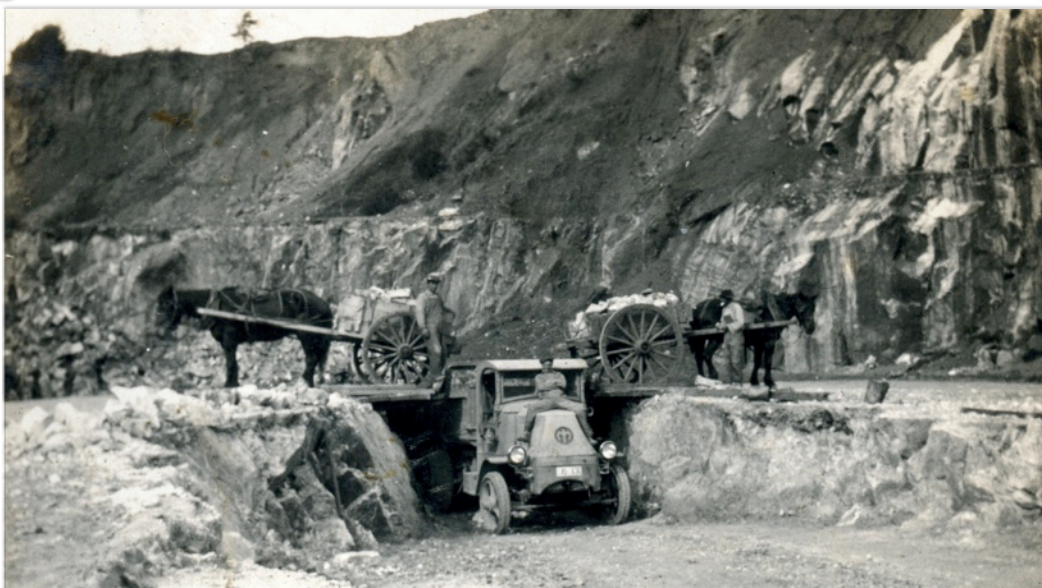
Scoop shovel and truck at the Rincon Quarry, 1920s. The shovel appears to be removing soil and other overburden that came down in a landslide.
