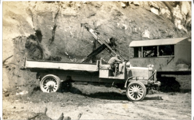
Scoop shovel and truck at the Rincon Quarry, 1920s. The shovel appears to be removing soil and other overburden that came down in a landslide.
