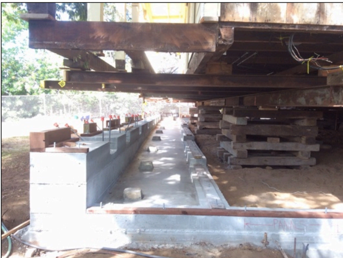
Above, original limestone rubble foundation under the Cardiff House. Below, new concrete foundation.
