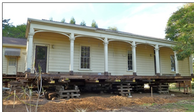
The Cardiff House jacked up off the ground in preparation for its new foundation.
