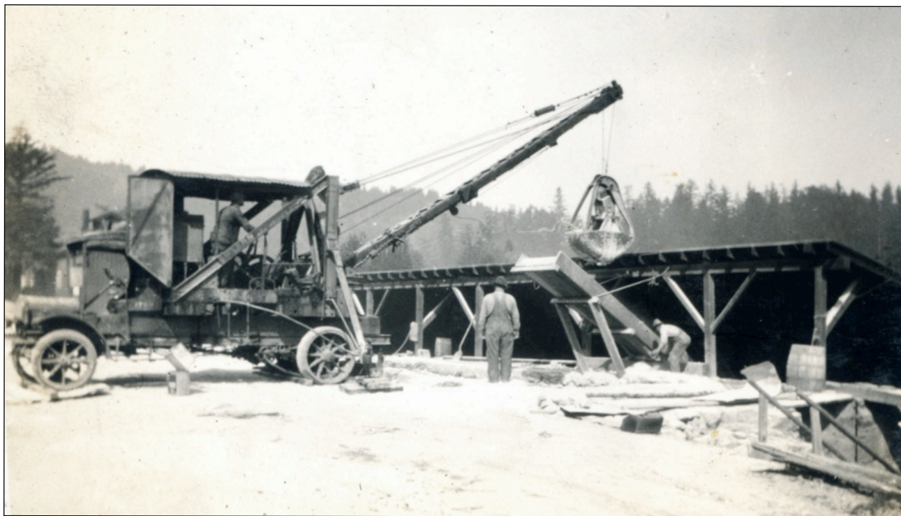
As technology changed, so did the methods for loading and unloading the kilns. This photo by George Silva from the 1920s shows one of the kilns at Rincon being unloaded by crane. Instead of removing the lime entirely from the bottom, some of it was lifted out at the top and dumped into a chute that directed it to the area in front of the kiln where it was put in barrels. (Wagner collection, Friends of the Cowell Lime Works Historic District)
