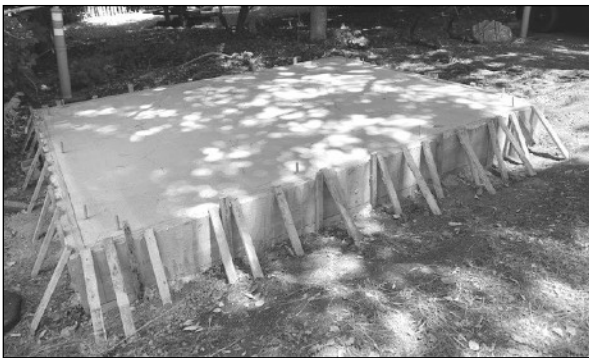
Concrete slab is poured.
