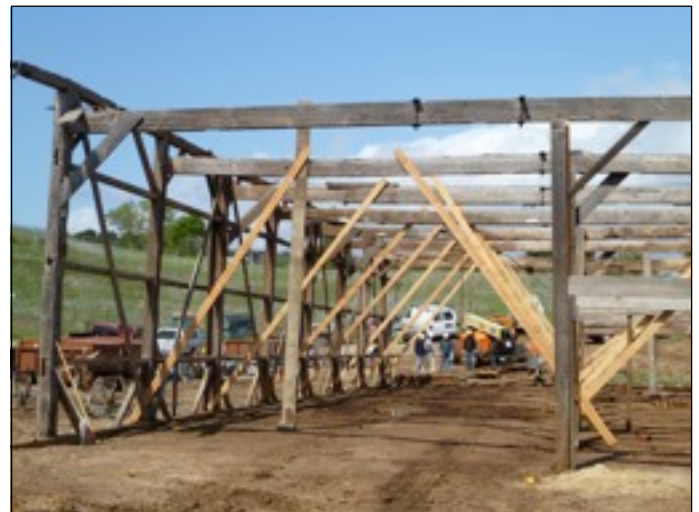
Temporary braces help hold the bents together until each is dismantled.
