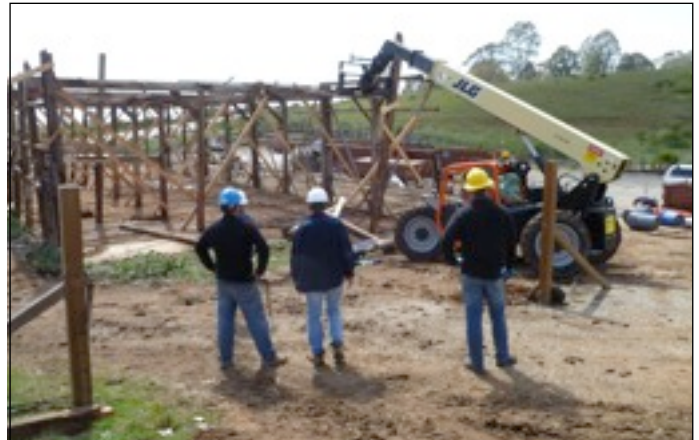
Dismantling a bent at the north end.
