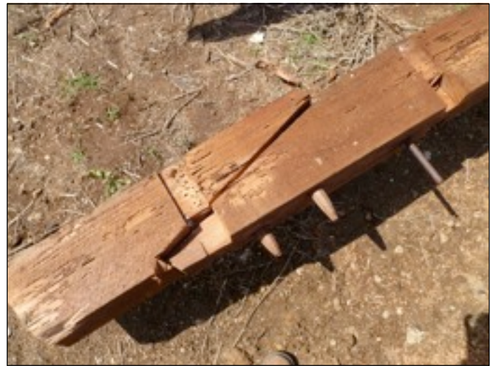
Section of ridge beam showing scarf joint and notches for rafters.
