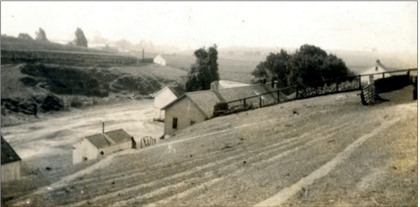
This view, probably from the late 1920s or 1930s, looks toward the southeast and shows the cook house (center). To the right is a garden, and nearby are several small buildings that no longer exist. Today's "Barn Theater" is on the far right. In the distance, just left of center, is a white building with a smokestack. This is probably the barrel mill, which burned before the University acquired the property. The smokestack was for a steam engine that ran a stave machine. (George Silva photo, courtesy of Barbara Wagner)
