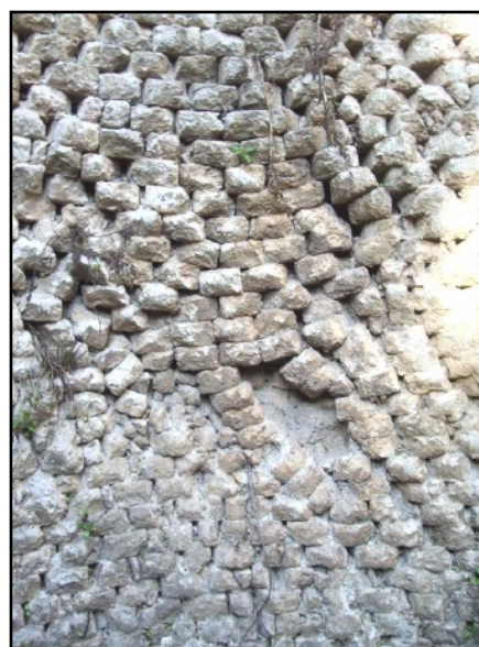
Portion of an interior kiln wall showing bricks badly damaged by the heat of the fires. Some bricks have been dislodged, and others have shifted position, giving a rather jumbled appearance.
