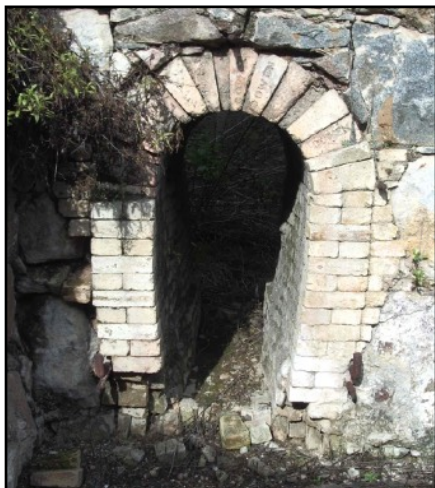
Each pot kiln has four doorways for inserting the wood fuel and for removing ashes and the finished chunks of lime. This one contains a mixture of COWEN and SNOWBALL bricks.
