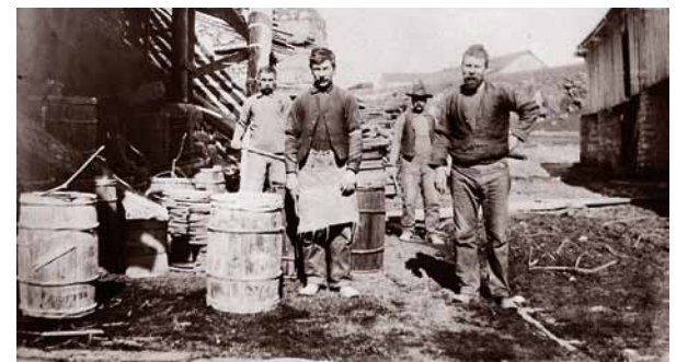
Kiln workers standing between cooperage (right) and kilns
